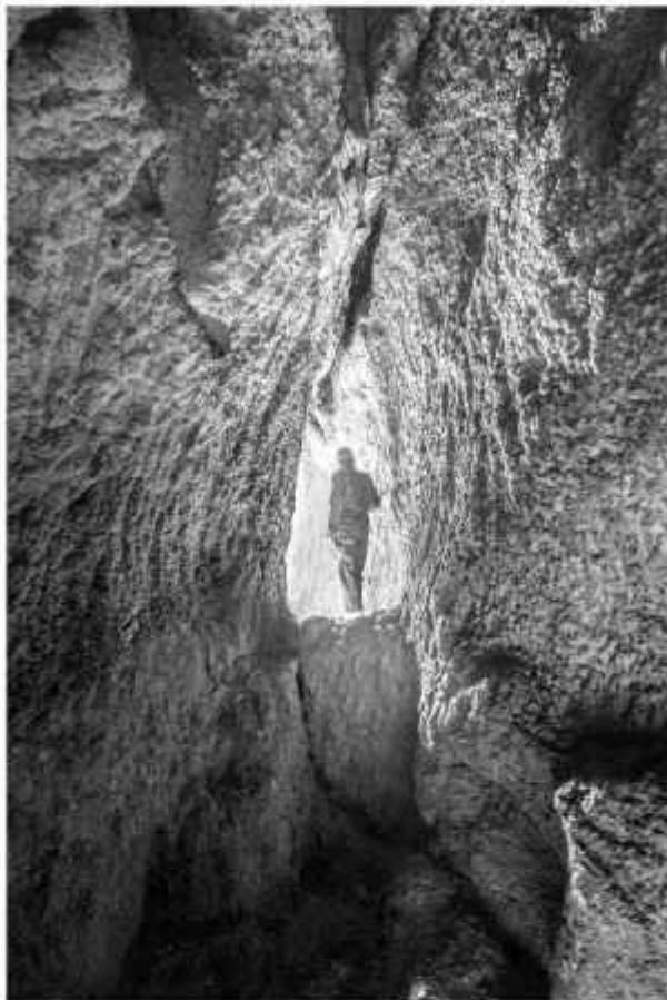
Fig. 4. The first part of Ca Toresina, the walls have many chisel scratches (Photo P. Lucci)
